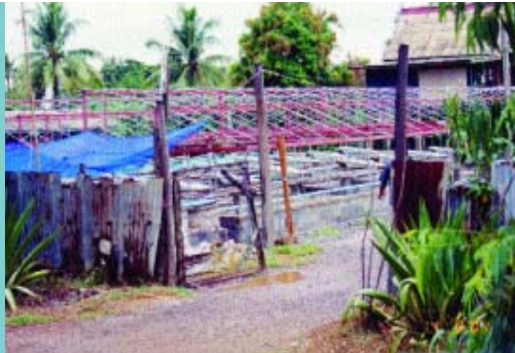
Figure 14c Buildings are often rebuilt as the hatchery prospers but the structure remains simple (Thailand)
