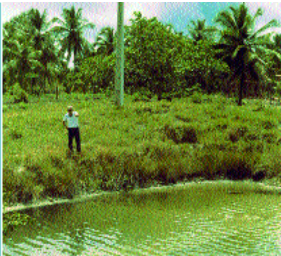
Figure 47 The bank of this freshwater prawn pond is being eroded because its slope is too steep (Hawaii)
