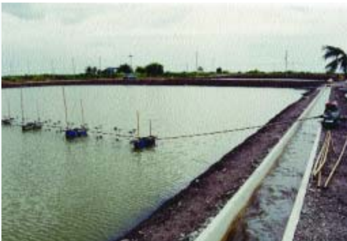
Figure 63 Power supplies are not always reliable. Loss of aeration at a critical time of the day and/or when ponds are heavily stocked. This Thai farm is using a mobile engine to drive long-shaft aerators in two adjacent ponds
